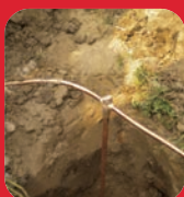
1. Copper bonded steel conductor, CBSC
